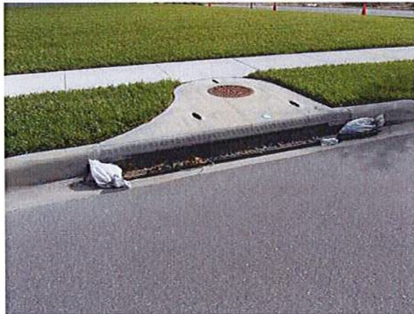
Typical catch basin at street
