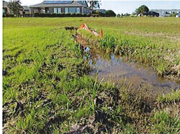
Accumulation of sediment at mitered end section control structure
