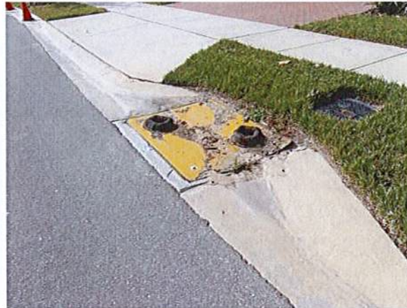
Typical catch basin at street
