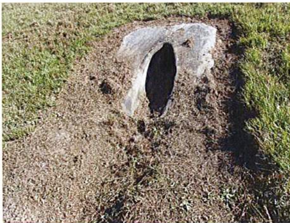
Mitered end section control structure
