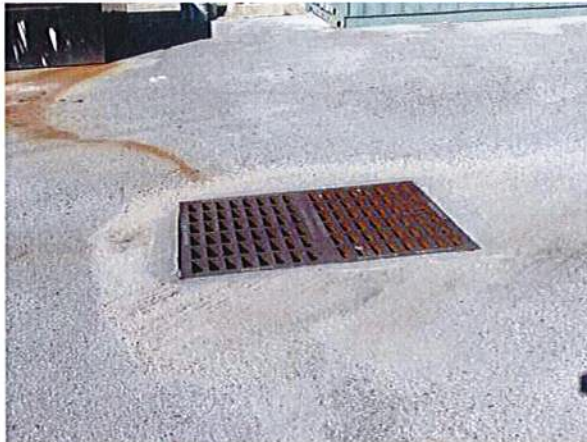
Typical catch basin at the clubhouse parking area
